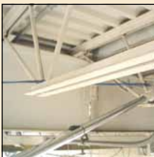
Ceiling Dust Removal
